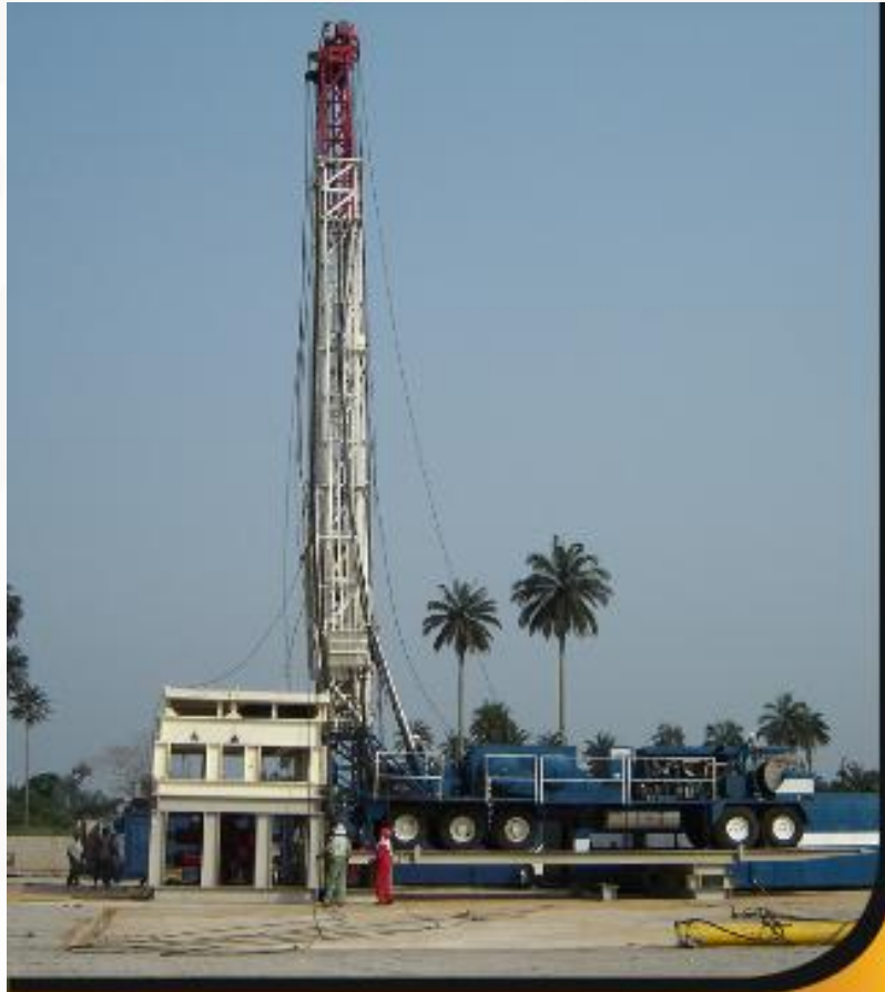
Compact NRG 101 service / drilling rig
